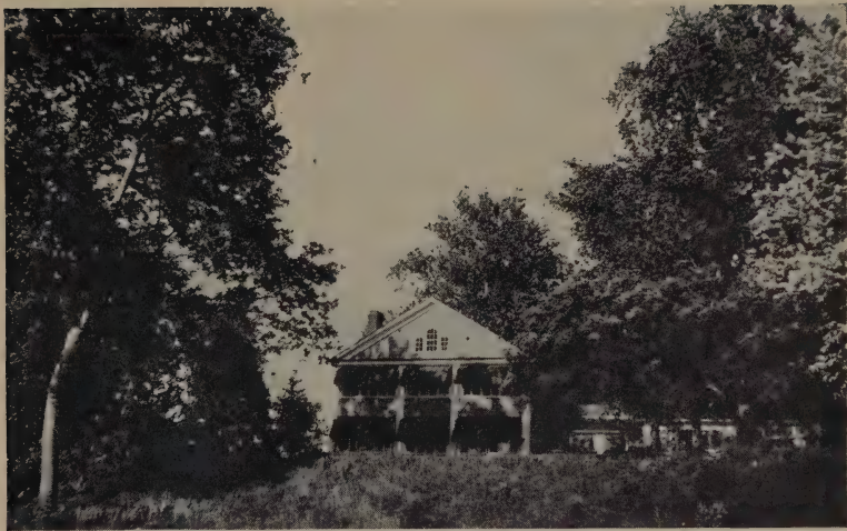
CHERRY HILL HOUSE BUILT BEFORE 1760
